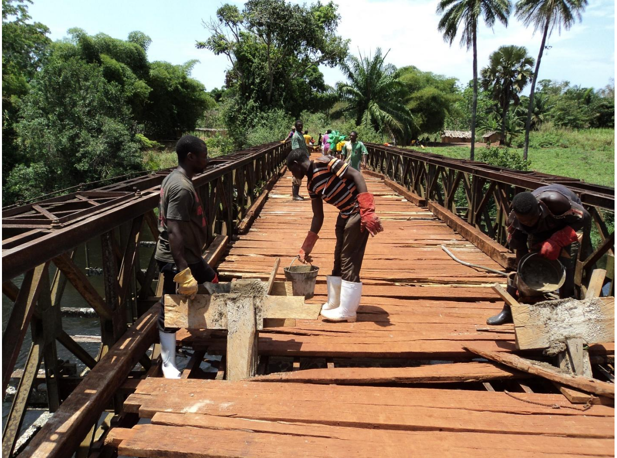
Bridge repair, DR Congo (© Medair)
