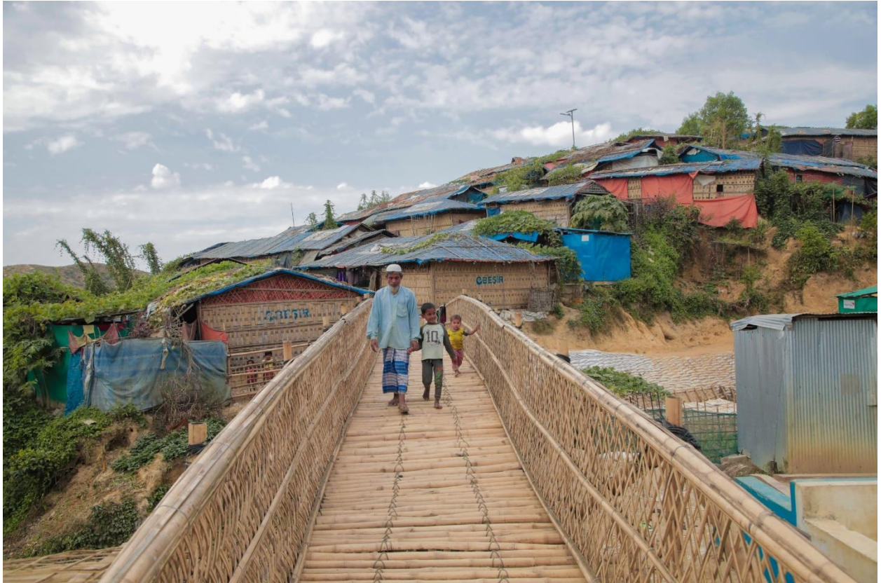
Bridge in Cox's Bazar Refugee Camp, Bangladesh (© World Vision)
