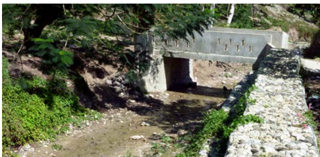
Structural river protection (Terre des hommes Foundation)
